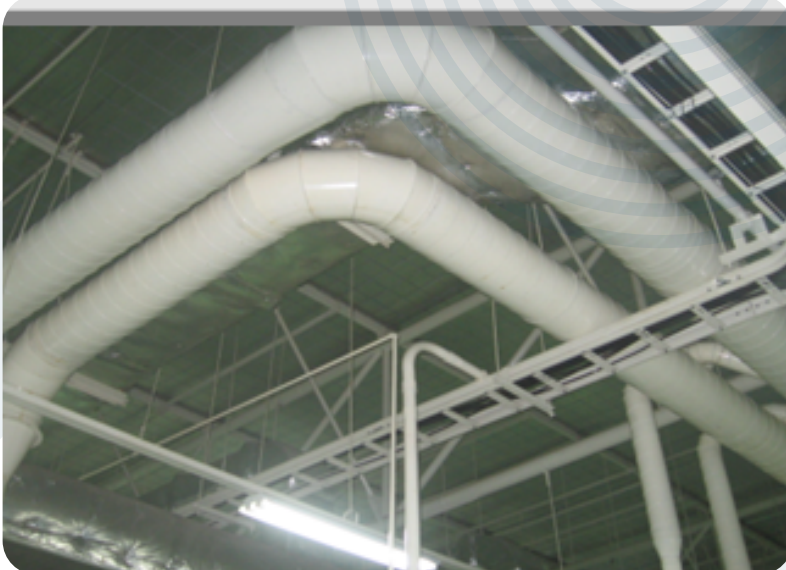
Spiral pipe installation work
