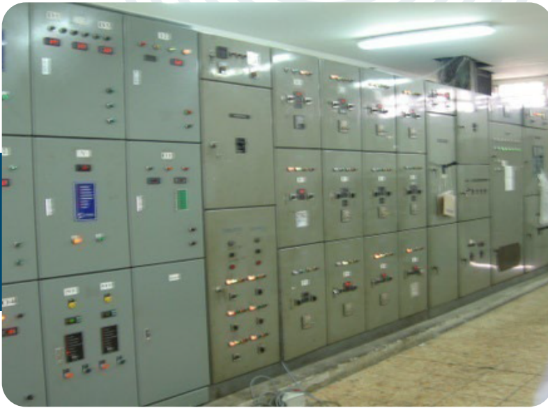
Install the Main Distribution Board cabinet
