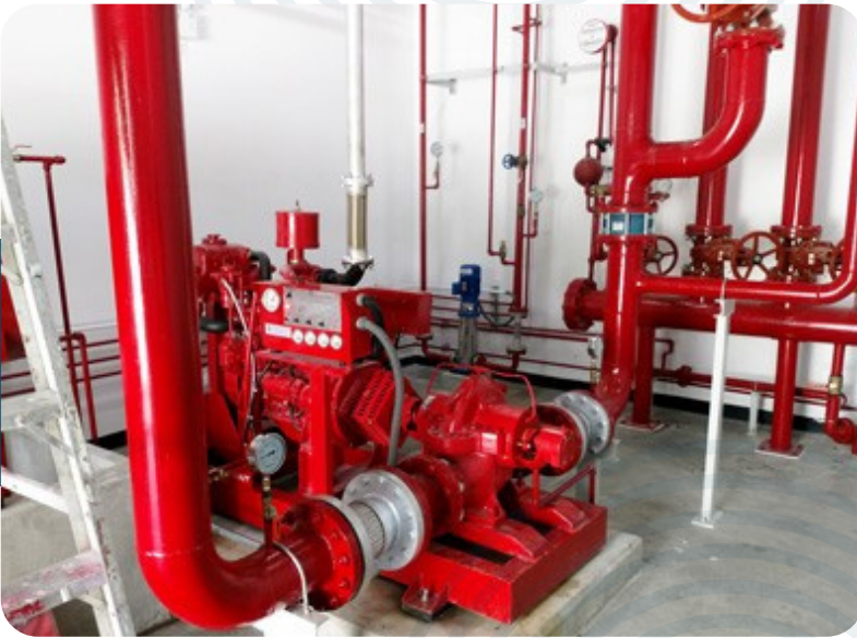
Fire pump system installation work
