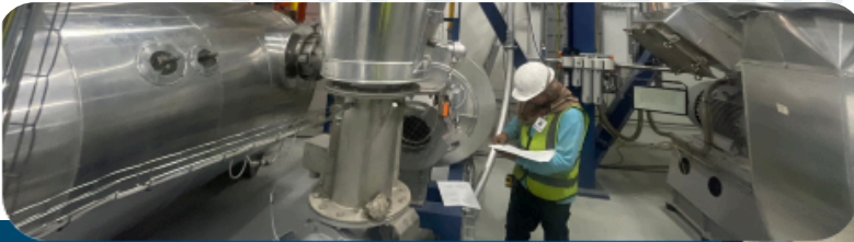
Aluminum jacket plate installation work
