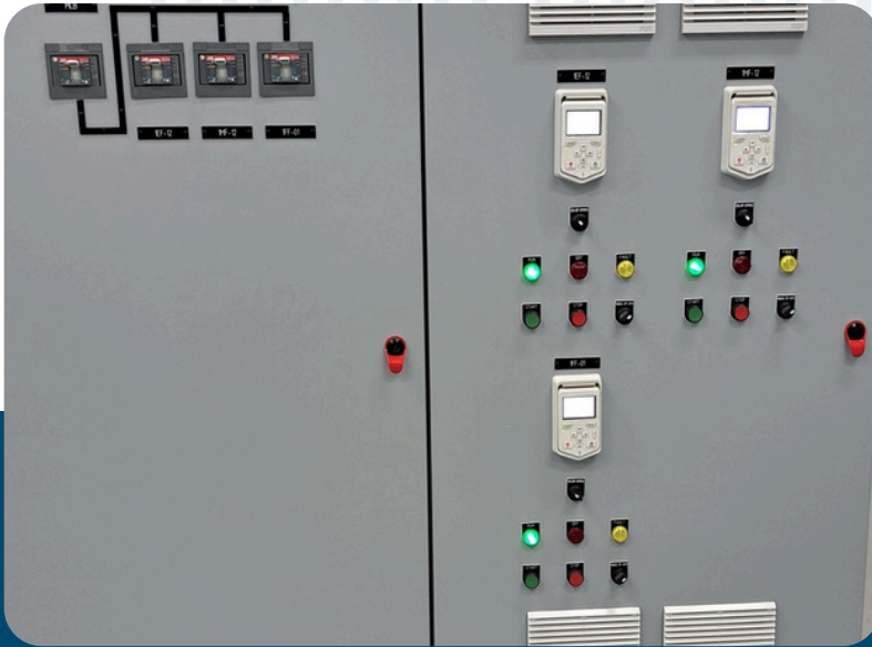
Install the Main Distribution Board cabinet
