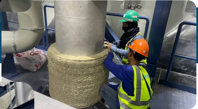
Thermal insulation installation work
